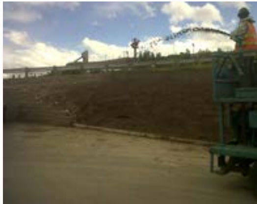
Biotic Earth is applied hydraulically, 2011.
